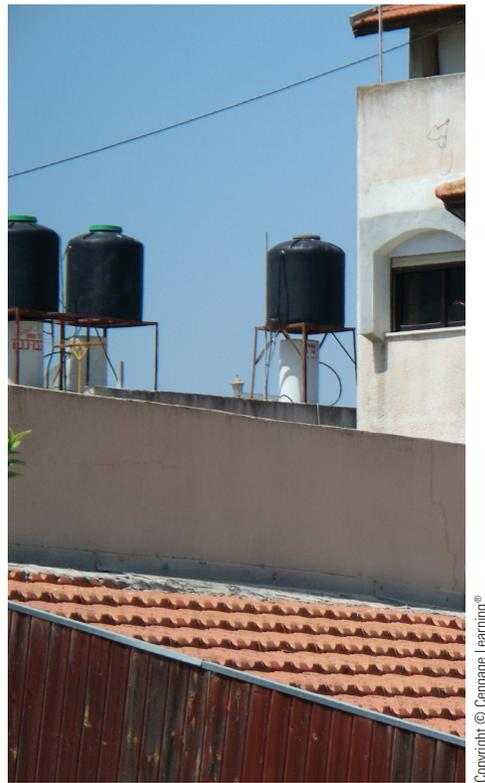
**FIGURE OCCUPATIONS 2** Solar water heaters mounted on a roof.
